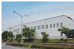
Kobe API Plant
